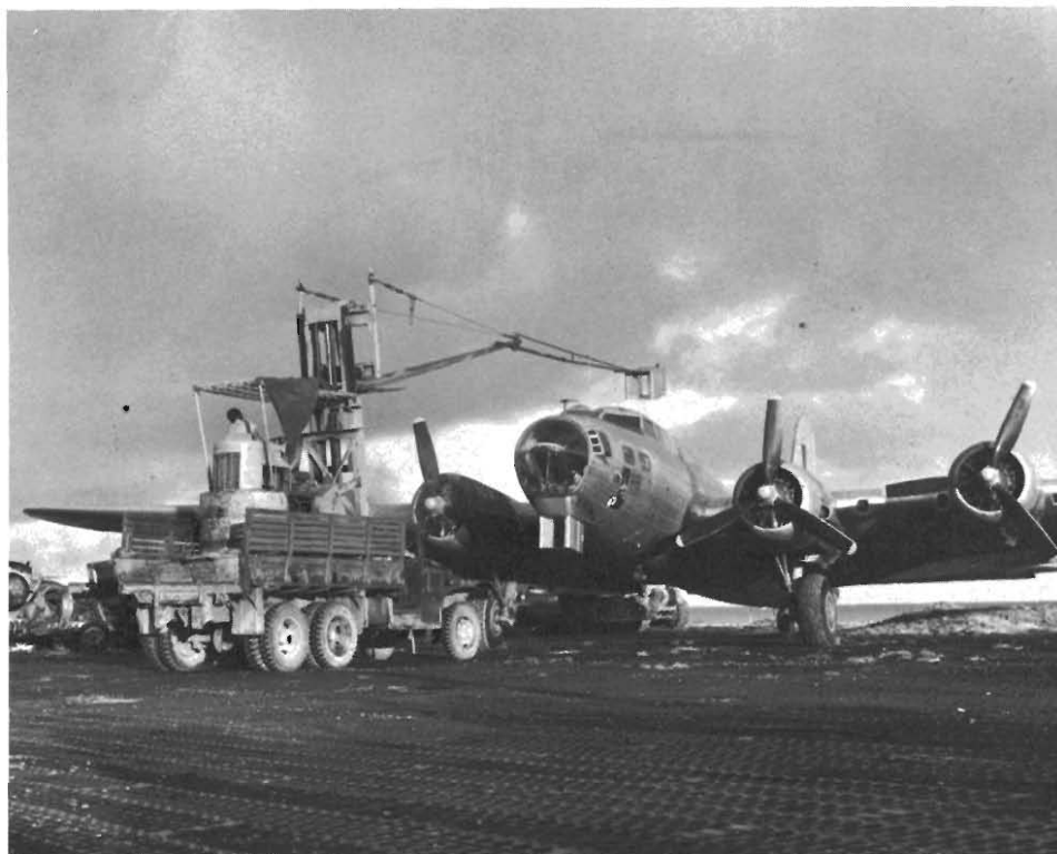
Samples of airborne debris from the Operation Crossroads tests of 1946 were gathered by drone aircraft. Shown here is a sampling unit being installed behind the cockpit of a drone B-17. The filter paper in the sampling unit was specially treated so that the debris would stick to its surface.
